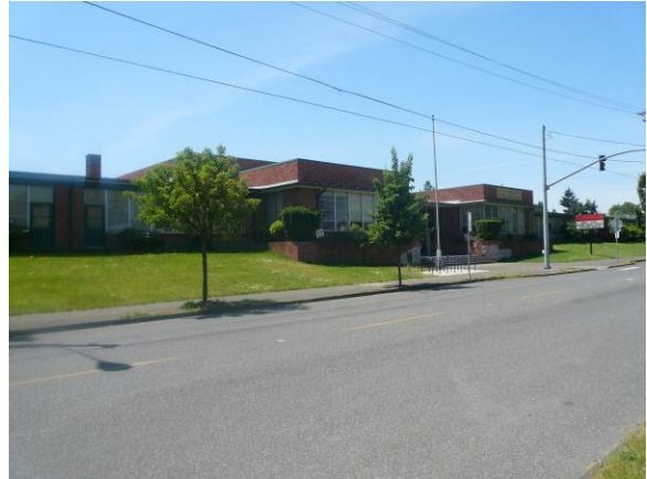
North elevation facing southwest
