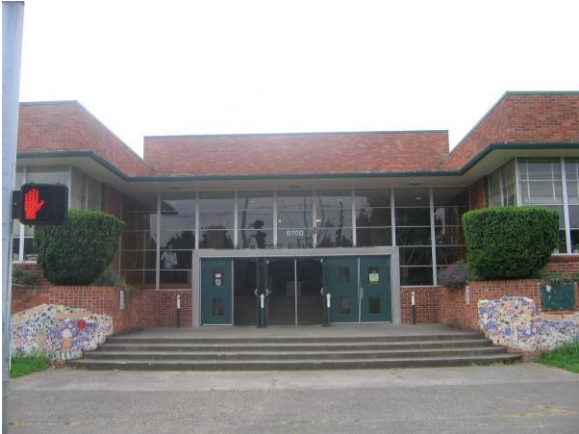
North elevation facing south
