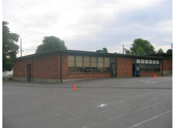
Addition facing southeast
