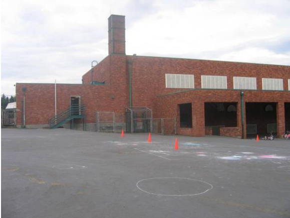
Southeast elevation facing southwest
