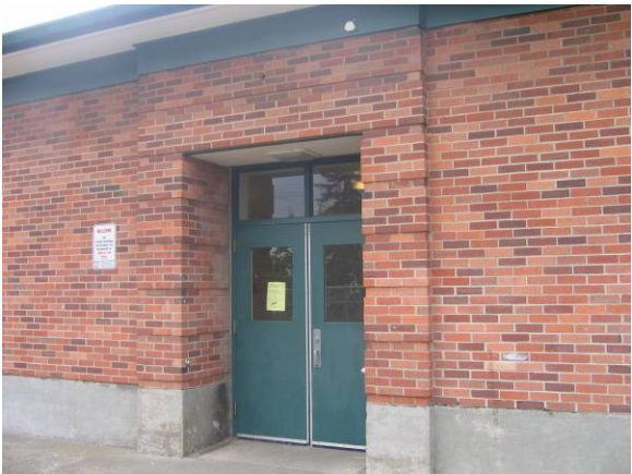
Brickwork facing north
